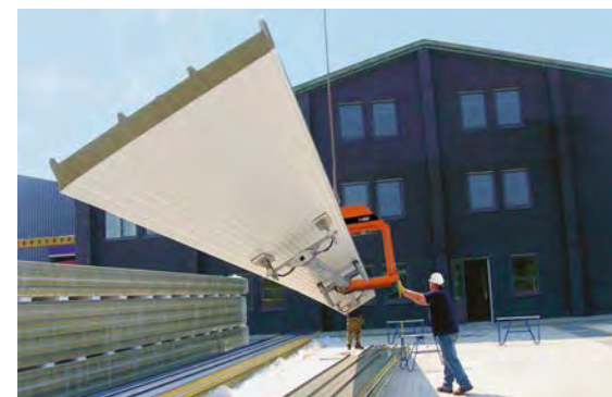
CladBoy Kompakt - easily rotates long roof panels.
