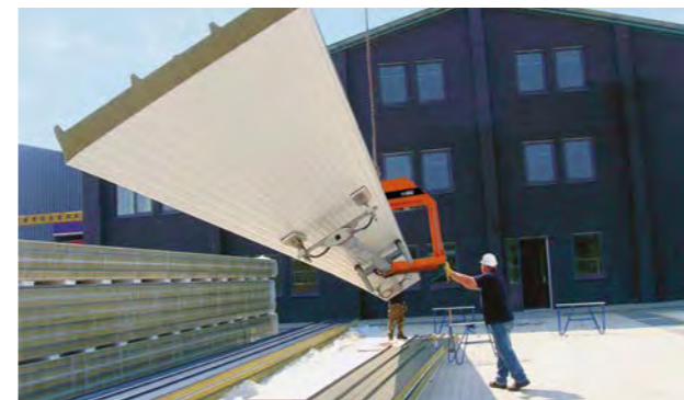
RotaBoy Kompakt - easily rotates large roof panels. Up to 350 kg. Please contact us if the weight exceeds 350 kg.
