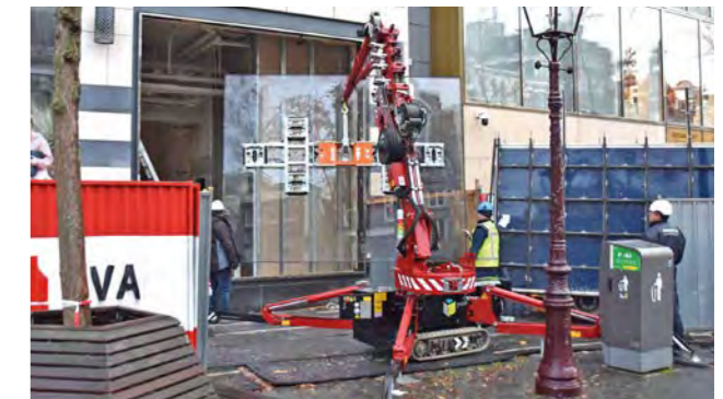
GBXL - all-round machine for installation of most glass elements up to 1,000 kg.
