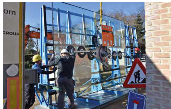
GBH - For large and heavy glass elements up to 1,800 kg.
